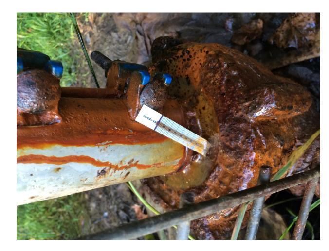
10-22-2018 Compliance Notice # 1536086906 follow up inspection. The injection line is disconnected from the injection tubing. The injection tubing has 64 psi. the compression clamp is located below the injection tubing master valve. The compression clamp is seeping brine out on to the wellhead slips and on to the ground.
