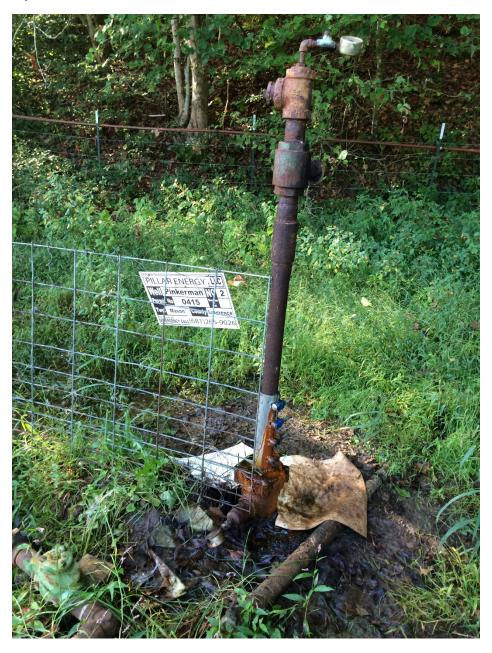
9-21-2018 Compliance Notice # 1536086906 follow up inspection. The injection tubing is disconnected from the injection line. The stainless steel clamp on the injection tubing is seeping brine onto the wellhead. A High Range Quantab was used to test the fluid on the wellhead ring. The fluid tested at more than 6907 ppm Cl. No contaminated soil has been removed from the location. The injection tubing pressure is 60
