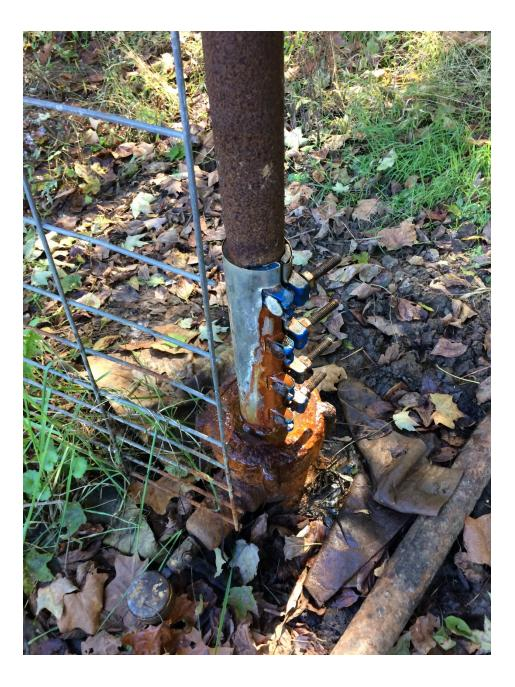
11-19-2018 Compliance Notice # 1536086906 follow up inspection. The injection line is disconnected from the injection tubing. The injection tubing has a compression clamp located above the wellhead slip ring. The compression clamp is seeping brine. The injection tubing has 70 psi. A High Range Quantab was used on the brine seeping from the clamp. The Quantab maxed out at more than 6907 ppm Cl.
