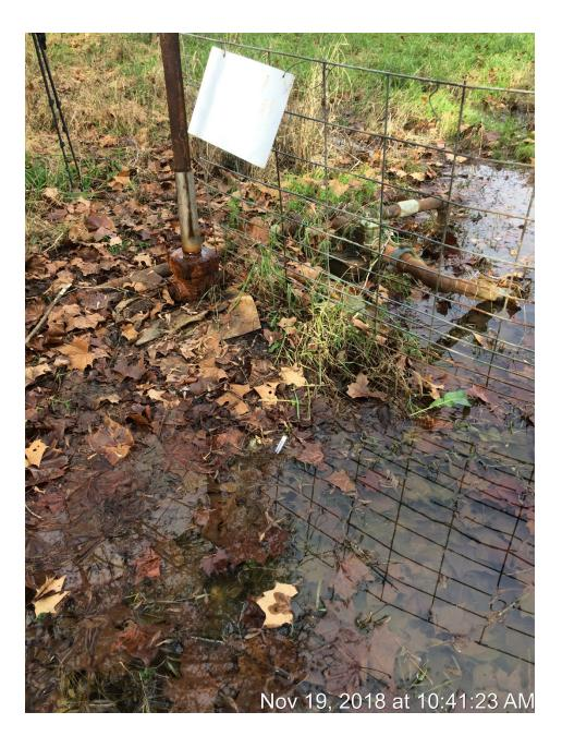
12-10-2018 Compliance Notice # 1536086906 follow up inspection. The injection line is disconnected from the injection tubing. The injection tubing has a stainless steel compression clamp installed. The compression clamp is seeping brine. The site is currently being used for cattle. The well does not have a fence around it.
