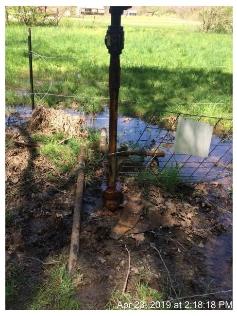
5-28-2019 Compliance Notice # 1536086906 follow up inspection. Brine is seeping from the hole in the injection tubing. The stainless steel compression clamp is not sealing off the brine leak. There is a 4 foot by 8 foot scald area at the well site. A 2inch steel plug has been installed in the 2 inch injection tubing master valve. The well site shows recent evidence of flooding with wood debris caught in the well fencing.
