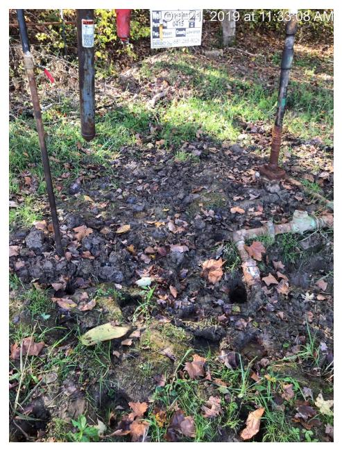
12-20-2019 Compliance Notice # 1536086906 follow up inspection. No contaminated soil has been removed from the location. The well site shows signs of recent flooding over the location including sticks, leaves and debris collected on piping and the wellhead. The annulus is frozen. The injection line valve and injection tubing master valve are open.
