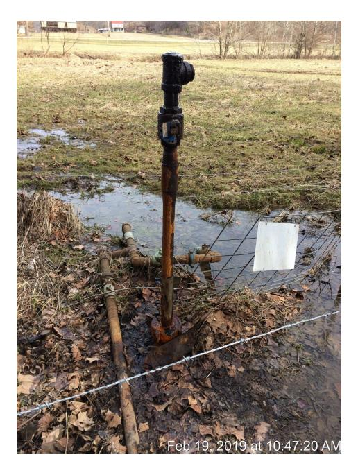
3-15-2019 Compliance Notice # 1536086906 follow up inspection. The well is disconnected from the injection line. The injection tubing is seeping brine from the hole in the injection tubing (between the wellhead slip ring and the injection tubing master valve.) The well is fenced in with barb wire and no access point to the well. Due to the fence, I was not able to install state issued pressure gauge to check the annulus pressure. The 1/4 inch fitting on the injection tubing has broken off.
