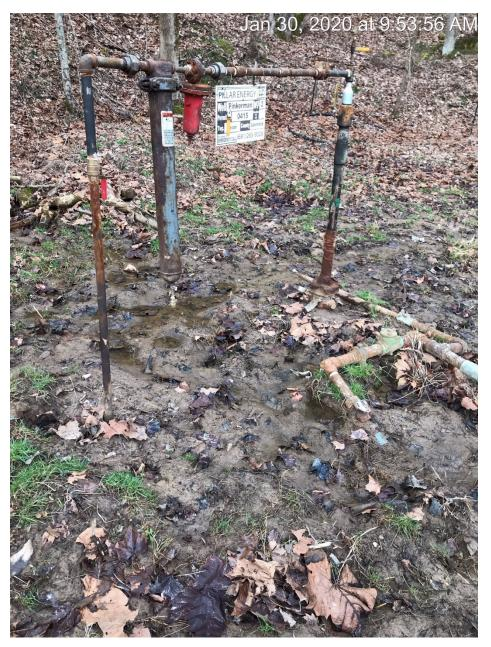
4-7-20 Compliance Notice # 1536086906 follow up inspection. Contaminated soil has not been removed from the location. Flood debris was observed at the well site from a recent event. Pictures were taken of the scald area.
