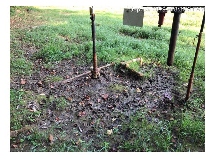
10-21-2019 Compliance Notice # 1536086906 follow up inspection. The access road gate was locked. Pillar well tender unlocked the gate. The injection line is connected to the injection tubing. All valves are open. Contaminated soil has not been removed from the well site. High range Quantab was used to test standing water at well site. Quantab result was 2840 ppm Cl.
