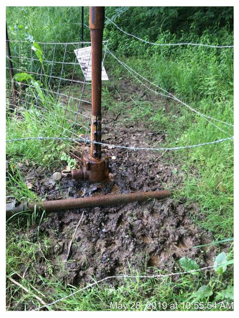
6-12-2019 Compliance Notice # 1536086906 follow up inspection. The injection tubing is disconnected from the injection line. The injection tubing has a stainless steel compression clamp that is located between the wellhead slip ring and the injection tubing master valve. The injection tubing is seeping brine onto the ground. The well site has a barb wire fence with no access point around the well.
