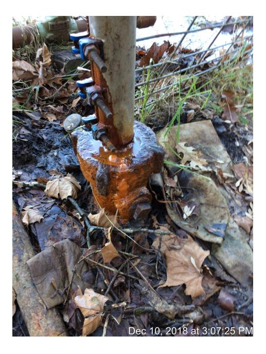
1-4-2019 Compliance Notice # 1536086906 follow up inspection. A barb wire enclosure has been installed around the well. The enclosure has no gate or access point. I was not able to install the state issued gauge and check pressures on the injection tubing and the annulus. The stainless steel compression clamp on the injection tubing was observed to be seeping brine.
