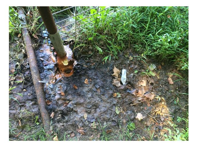
9-14-2018 Compliance Notice # 1536086906 follow up inspection. The injection line has been disconnected from the injection tubing with both ends plugged off. The stainless steel compression clamp is showing signs of leaking, orange stain running down to the ground. Absorbent pads have been placed on the ground recently. No contaminated soil has been removed from the location. Identification is posted.
