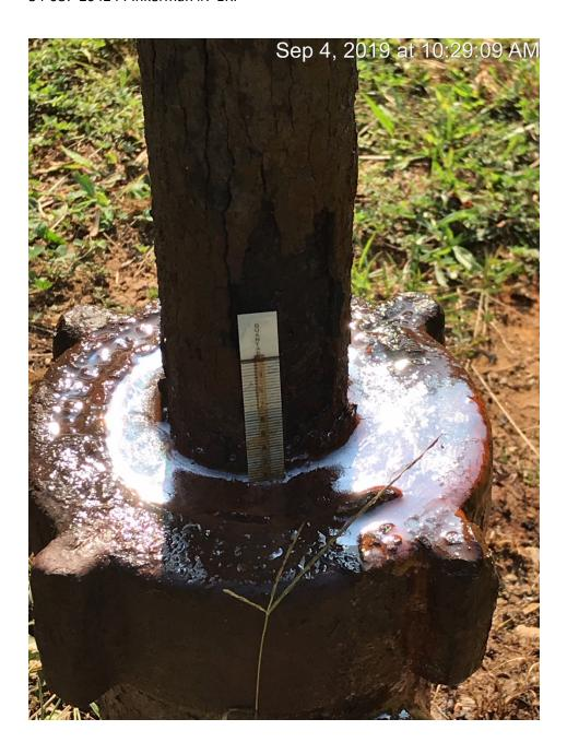
9-13-2019 Compliance Notice # 1567619883 follow up inspection. The injection line valve is closed. The injection tubing master valve is closed. The injection tubing insulation and scale have been removed. The tubing is wet but not currently seeping brine. The scald area is 24 inches by 24 inches.
