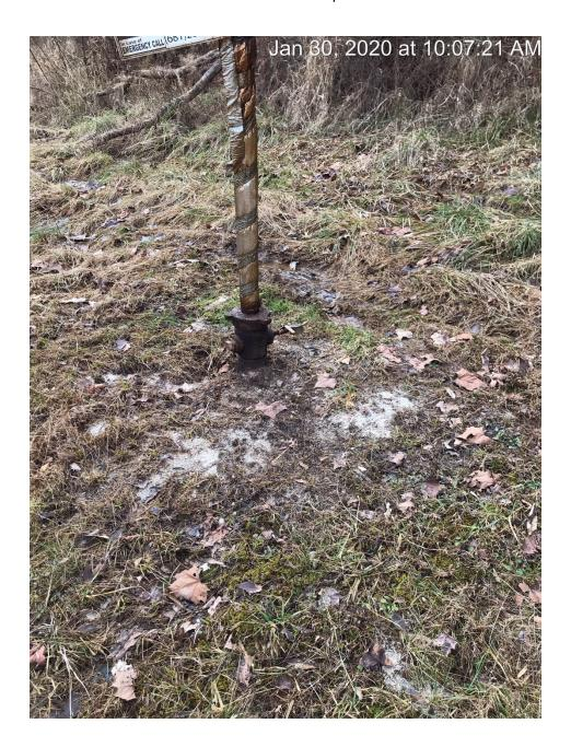
4-7-20 Compliance Notice # 954126558 follow up inspection. Contaminated soil has not been removed from the location. Grey absorbent material is still coating the ground around the well. A black plastic bag with contaminated material is on location.
