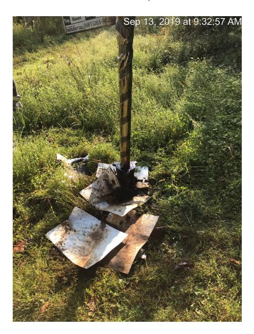
10-21-2019 Compliance Notice # 954126558 follow up inspection. A 6 foot by 4 foot area at the wellhead has absorbing material applied to the ground. A black plastic bag is on site with contaminated material and used absorbing pads in it. No contaminated soil has been removed from the spill site.
