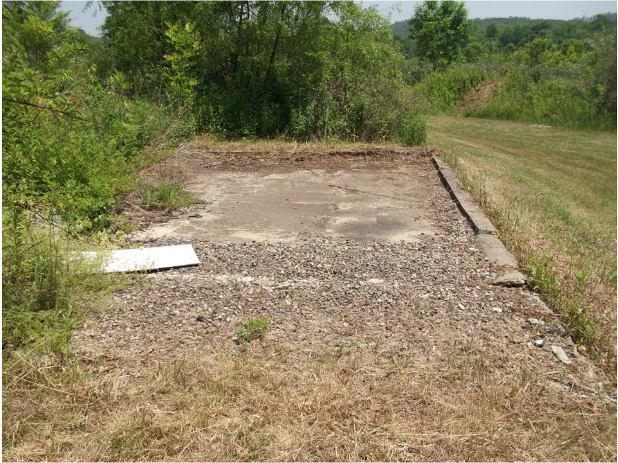
This photo shows the unloading pad for the Adams Oil and Gas Enhanced Recovery Injection well 34-163-20318. Photo taken on 6-10-15 By ODNR/DOGRM UIC Inspector Jon Scott.
